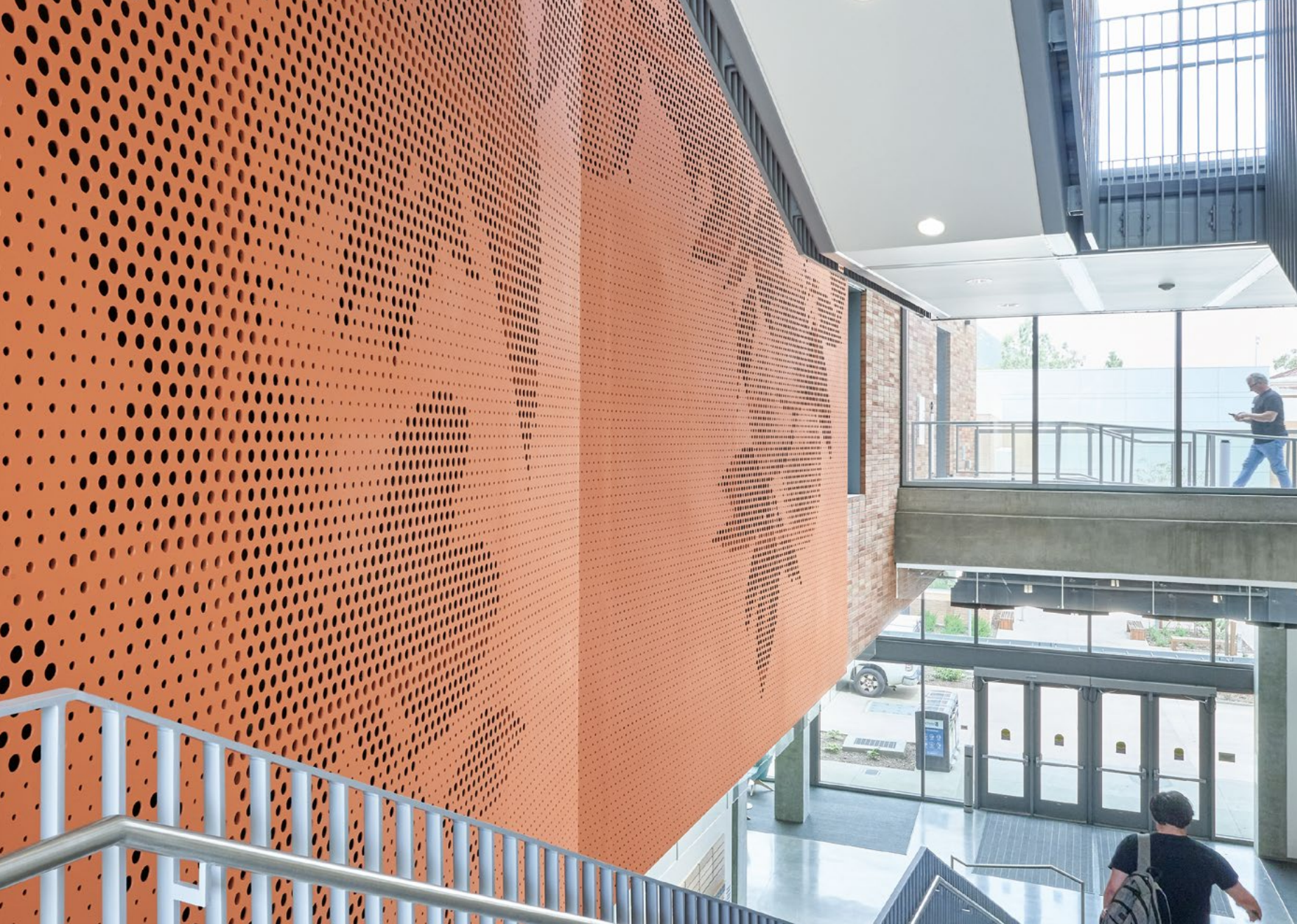
Custom CastWorks™ GRG walls UC Riverside School of Medicine Hensel Phelps, CO Architects
